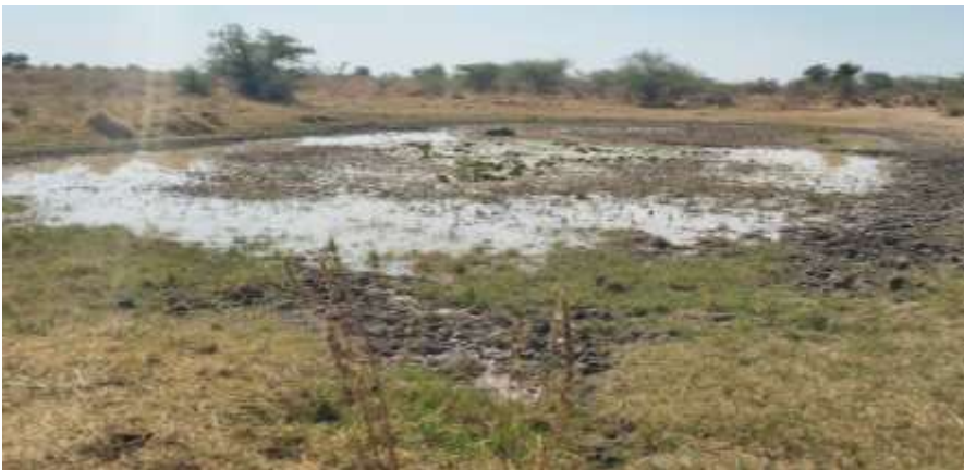
Poor governance of water catchment of dams, leading to high siltation and insufficient water storage for the community during dry spell. This situation, requiring intervention to increase adaptation of community to water scarcity.
